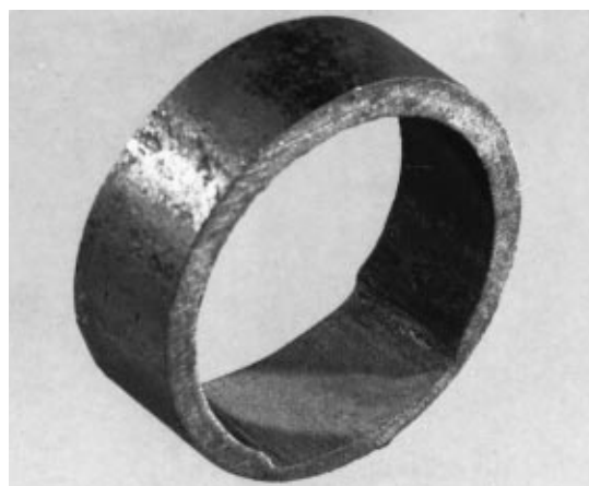
Figure 1 — Carbonic acid attack on condensate piping
